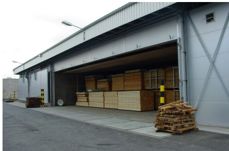
Fig. 2 Industrial kiln for pre-drying, drying and conditioning of timber during heat treatment
