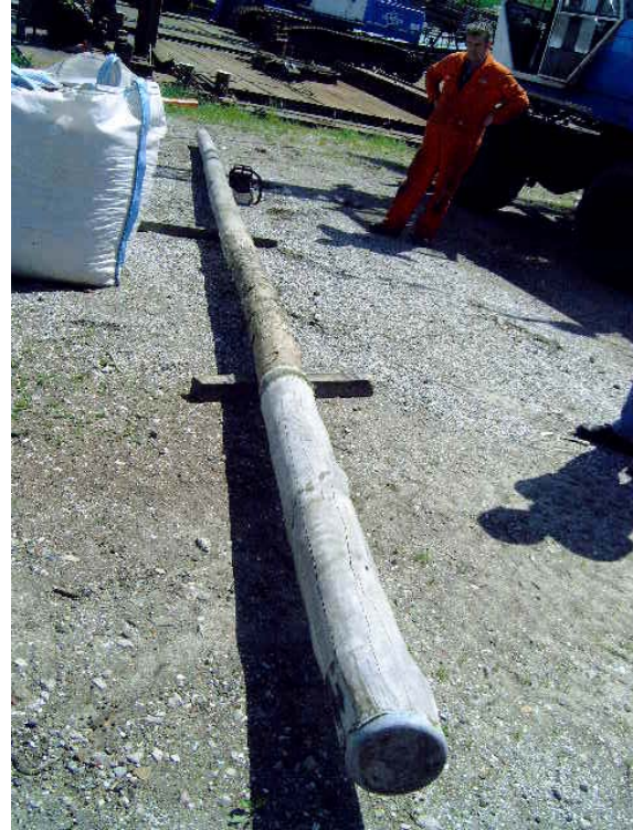
The investigated pole, after being taken out
